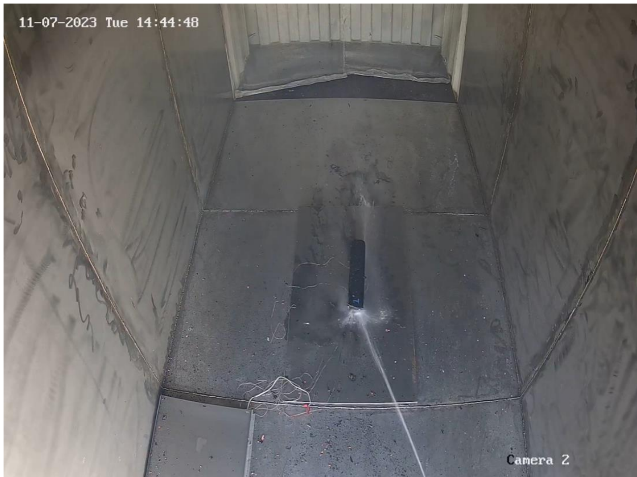
Figure 84. End of application of FCL FSS.
