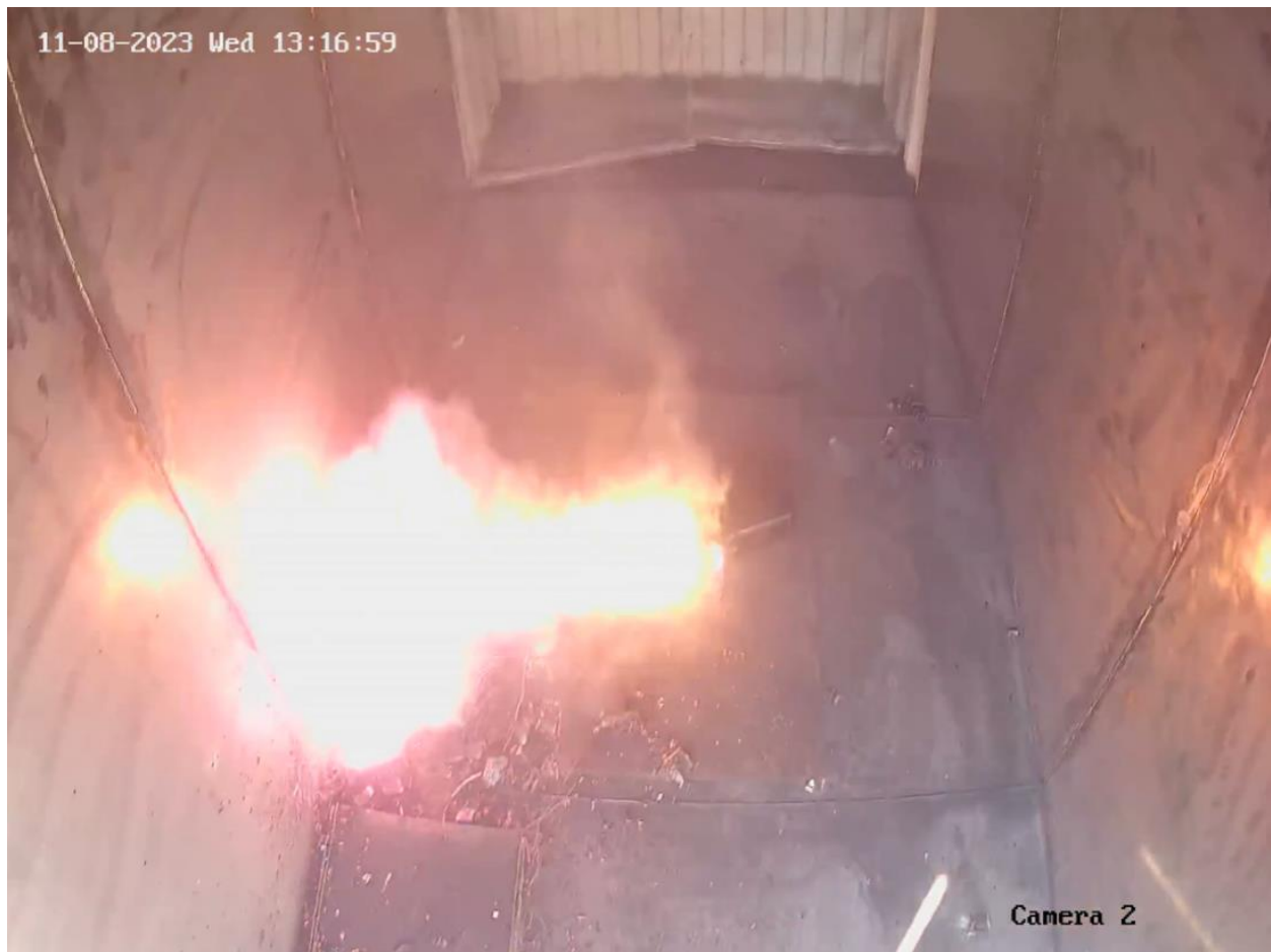
Figure 96. Progression photo of control battery experiencing thermal runaway.
