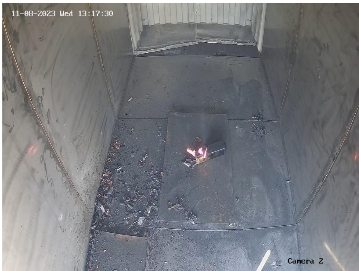
Figure 97. Control battery begins to move from force of cells going into thermal runaway.
