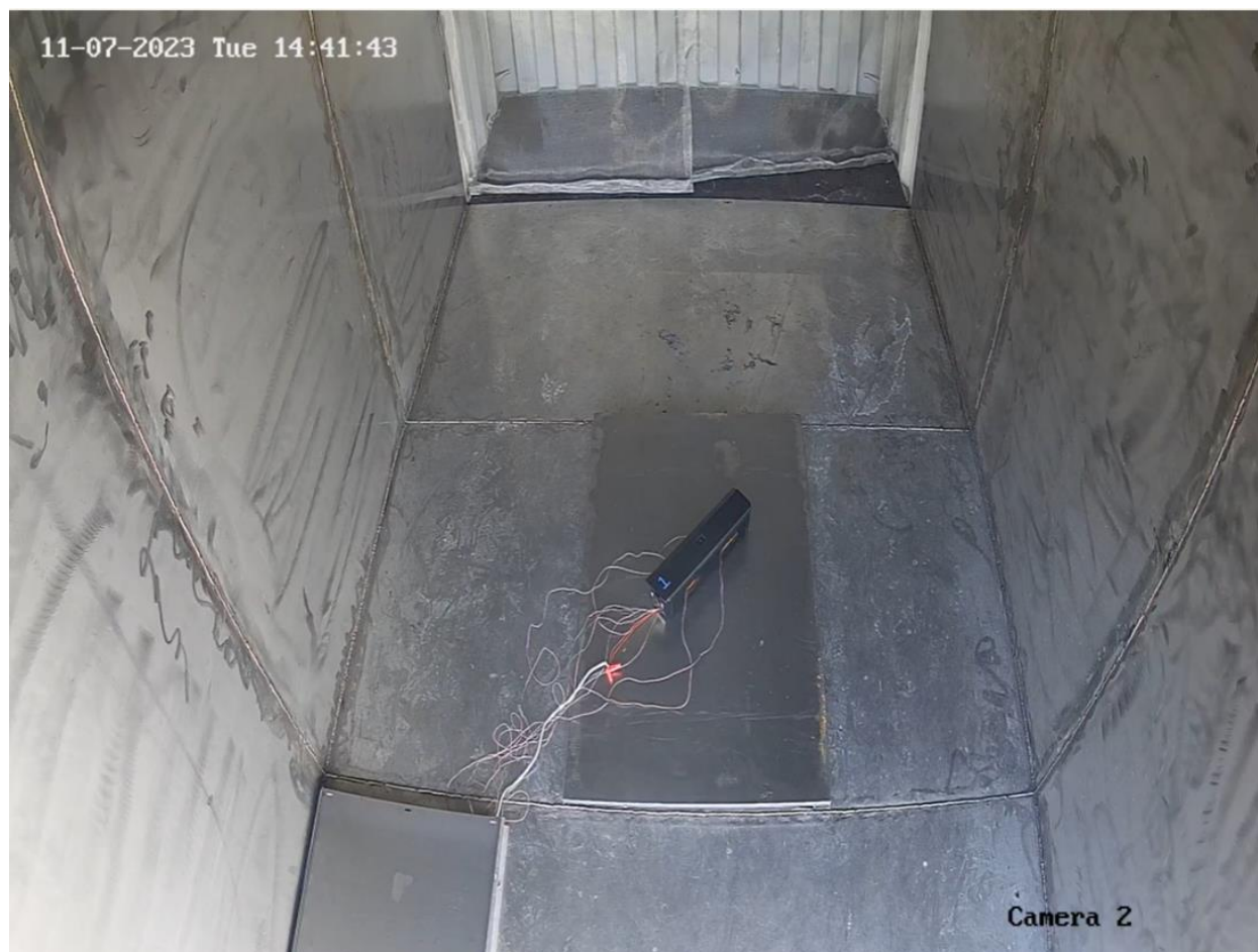
Figure 78. View immediately before the first cells experienced thermal runaway.
