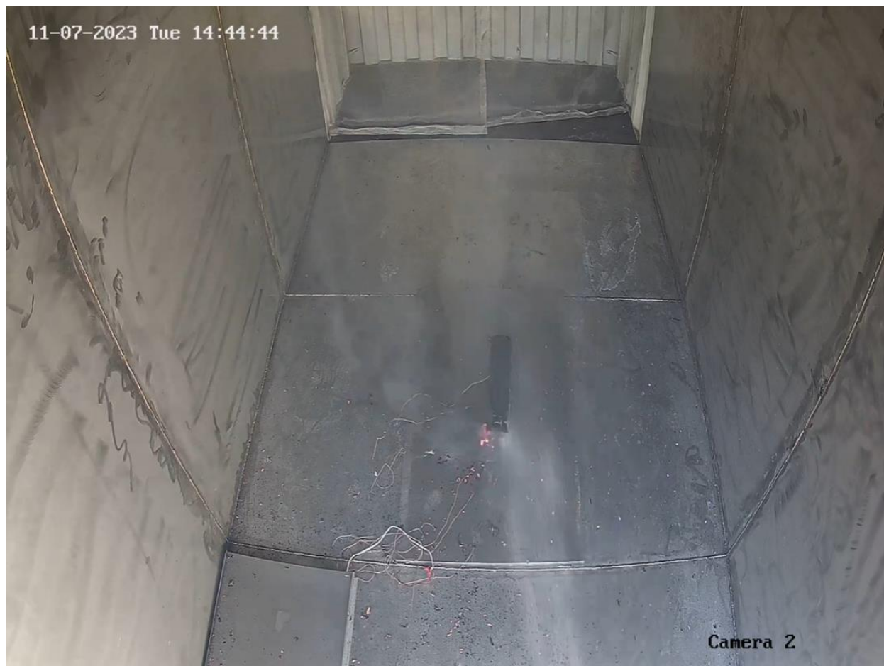
Figure 83. Start of the application of FCL FSS.
